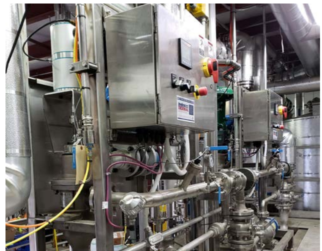
Photos provided by MPC Group showing installation of Hydro-Thermal EZ Heater skids
